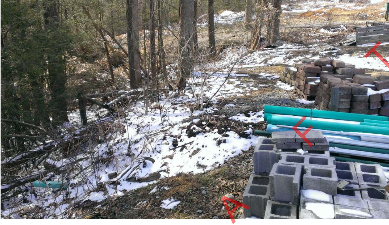
Block and pipe stored at the Cemetery site.
